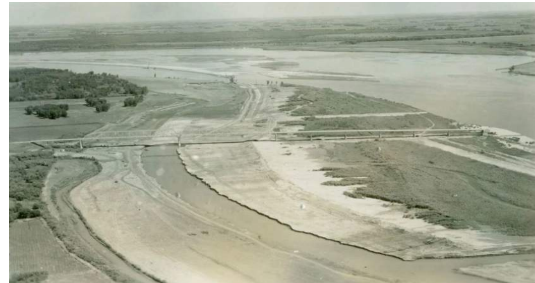
Photo: Partially completed bridge & USACE excavation, 1955.
