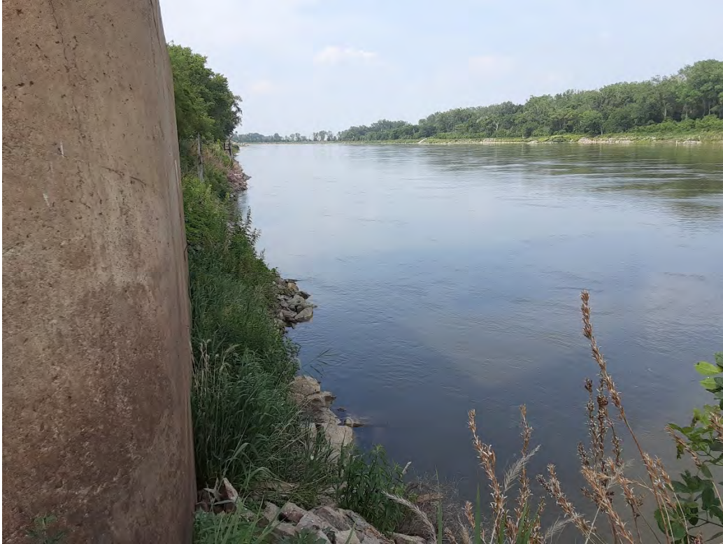
On Bank at Pier 1, Looking Upstream.
