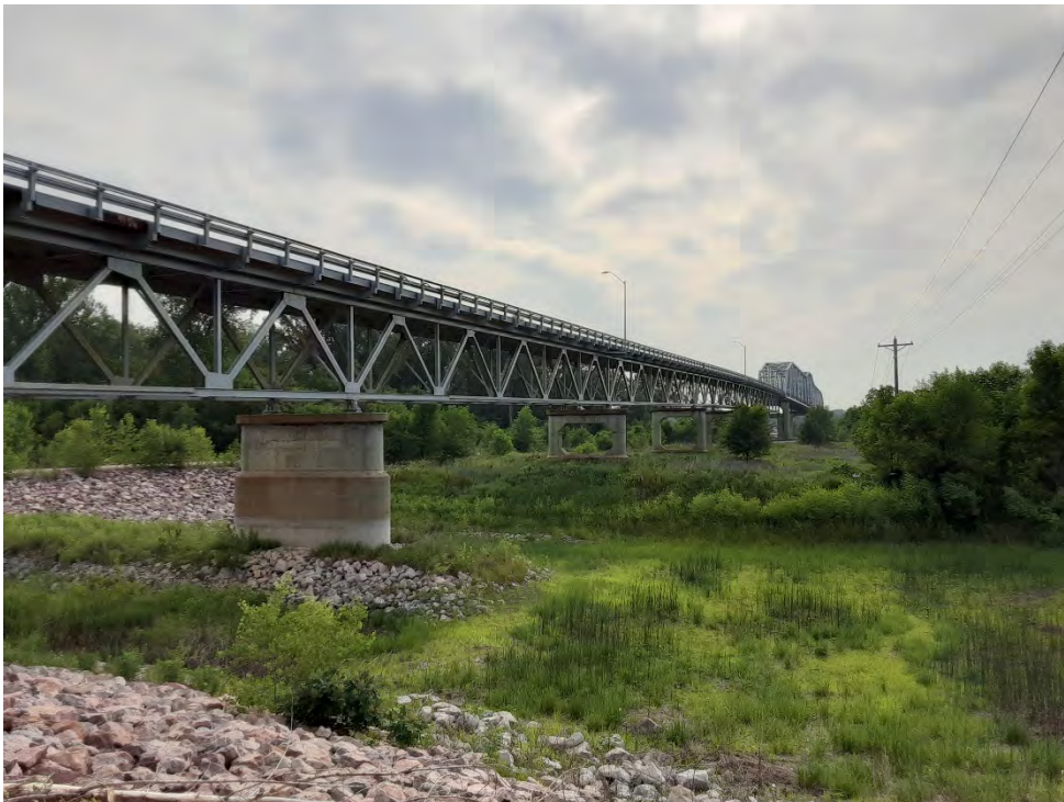
Iowa Approach Span, Looking Southwest
